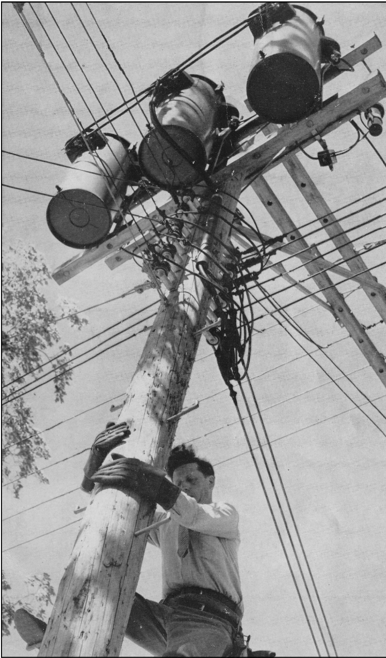
George coming down a pole after replacing a transformer fuse.
