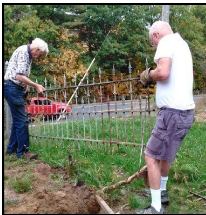
Larry and Terry carefully removed the bolts between the eight foot sections to prevent any damage to the fence. It would be interesting to know how old this fence is.
